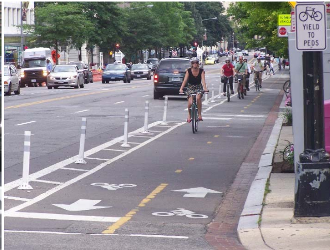
Left: a one-way cycle track protected by a parking lane and buffer and showing optional green paint. Right: a two-way cycle track, protected with optional flexible bollards and buffer.
