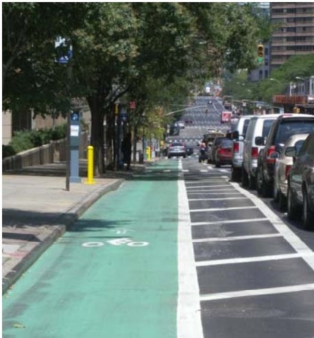
Left: a one-way cycle track protected by a parking lane and buffer and showing optional green paint. Right: a two-way cycle track, protected with optional flexible bollards and buffer.
